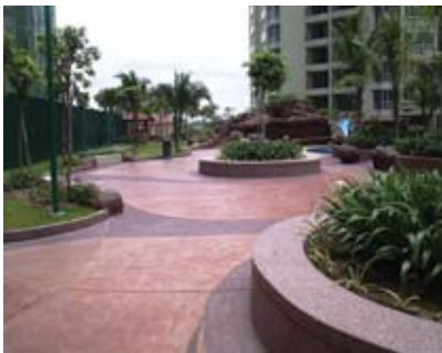
Masterpav Concrete Imprint to Condominium
