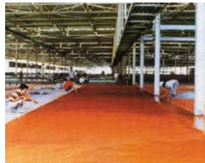
Silica Quartz Floor Hardener to Factory
