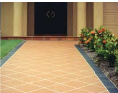
Masterpav Polymer Floor Texture to Bungalow
